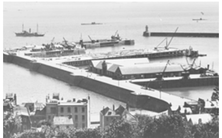
The harbour from the Blue Mountains in 1927. The deck of the jetty virtually complete but the buildings not yet started.
